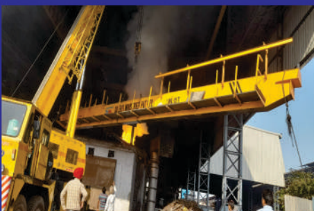
EOT CRANE - DOUBLE GIRDER - ERECTION AT SITE
