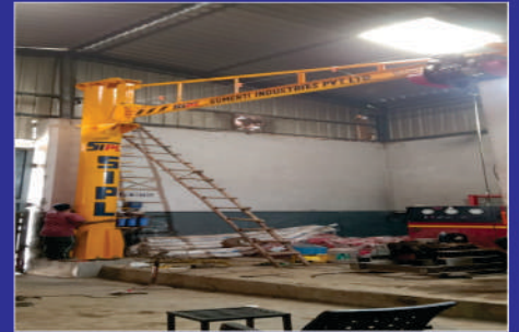
JIB CRANE - UNDER INSTALLATION
